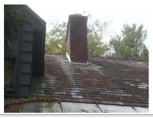
Observed chipped slate on eaves. This allows rain water to hit and infiltrate the wood trim below. Recommend qualified contractor repair.
