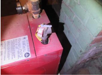
The average life expectancy of a gas boiler is about 15 years. The boiler in the home appears to be older than that. Recommend that this system be serviced every two years by a qualified heating and cooling technician. Recommend budgeting for a replacement in the future just in case.
