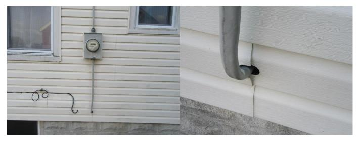
Observed loose siding panels that have pulled away from the exterior wall. This can allow rain to penetrate the wall and is susceptible to wind damage. Also observed a missing section of siding and other small areas of damage to the siding and trim that can allow water to penetrate the wall. Recommend qualified contractor repair.
