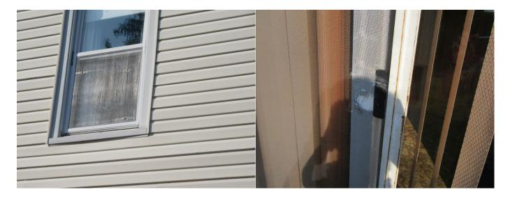
Observed gaps in trim and window wrap around windows. Observed a small amount of wood rot of window seal where gap was present. Recommend qualified person seal all gaps to prevent further water damage.
