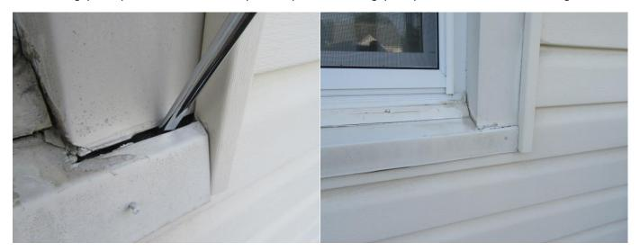
Observed damage to metal trim around garage overhead door. Trim is still functional to keep the weather out. Recommend repair if desired for cosmetic reasons.
