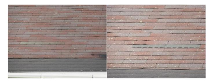
Observed presence of lichen growth on roof surfaces. While this is not expected to have much impact on the roof life, it does alter the appearance. Recommend contacting qualified roof cleaning contractor if desired to be removed.
