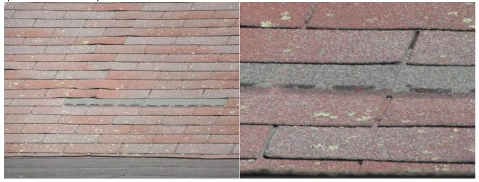
Observed lifting of shingles. This does not appear to affect the function of the roof covering. However, lifting of shingles can be caused by high temperatures in the attic space below. Excessive heat in the attic can shorten the life of asphalt shingle roof coverings. Lifted shingles are also more likely to suffer from wind damage. Recommend monitoring roof covering for loose or lifting shingles going forward.
